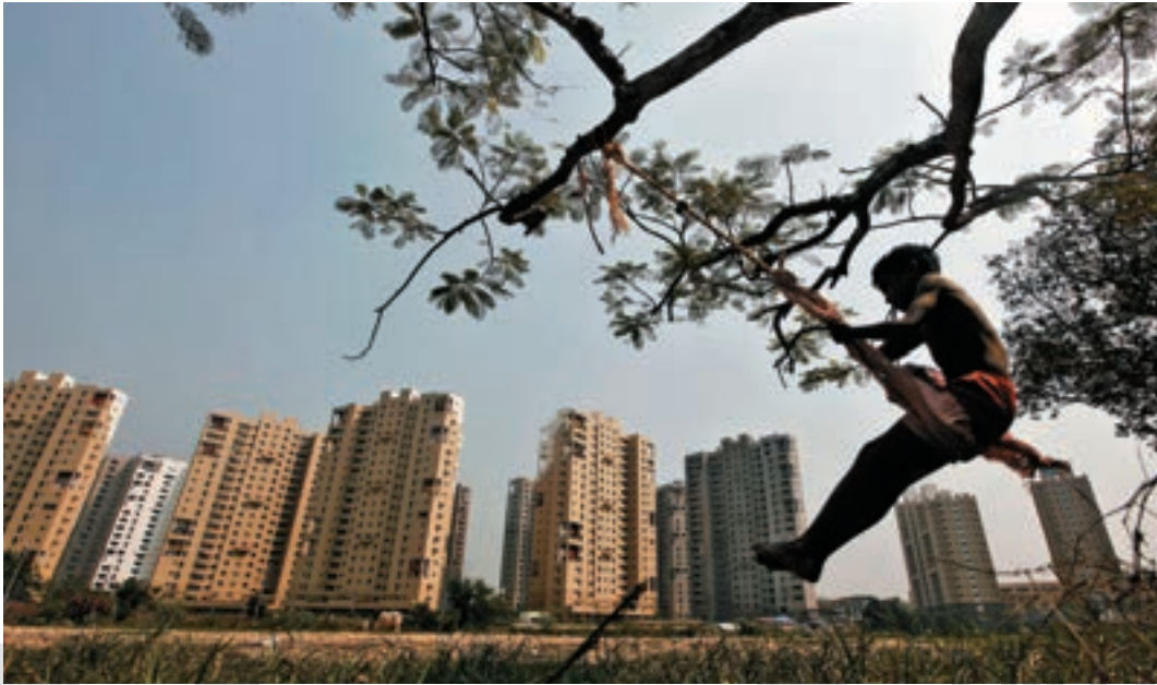
A residential estate under construction in Kolkata. Today we have a once-in-a-lifetime opportunity to use urbanisation to set off a virtuous spiral of social and economic development
